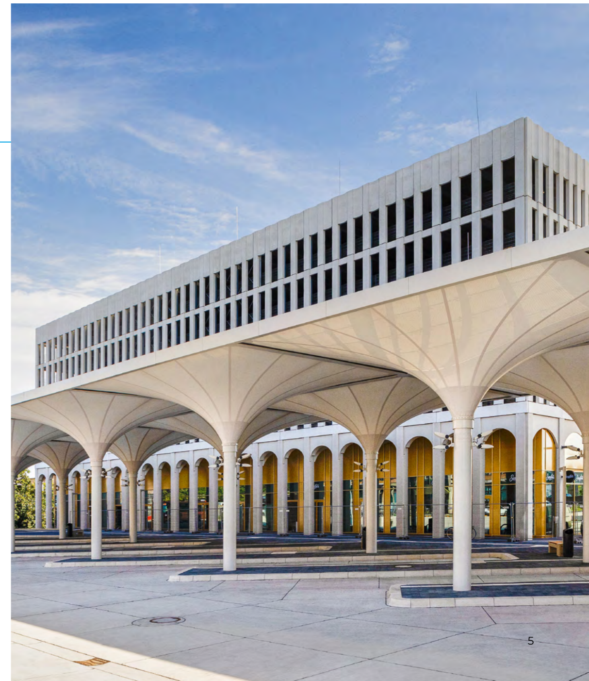
Intercity bus terminal Bremen with approx. 500 parking spaces on 15 levels
