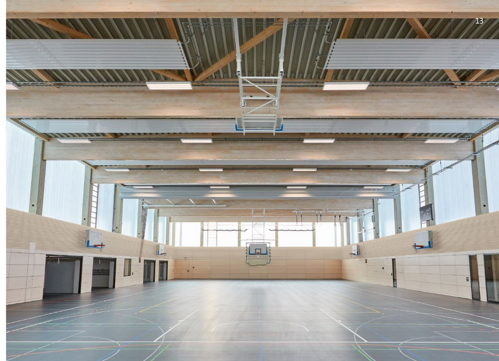
Sports hall with glulam timber beams in Düsseldorf.
