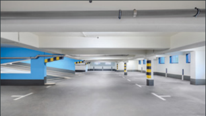
After existing building refurbishment
