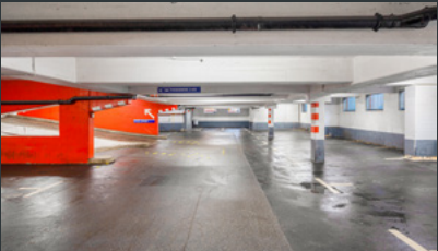
Before existing building refurbishment
