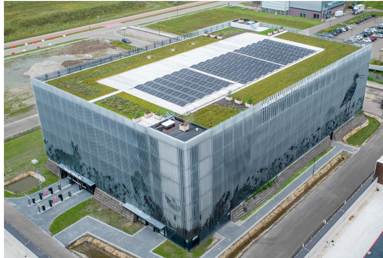
University of Leiden, Leiden, Netherlands, six levels, 430 parking spaces
