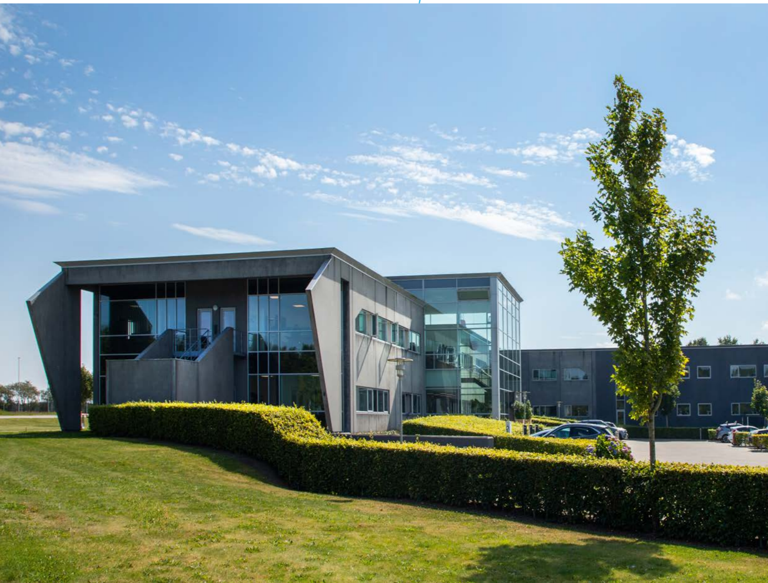
Eurowind Energy A/S, Hobro, Denmark, 1,107 m 2
